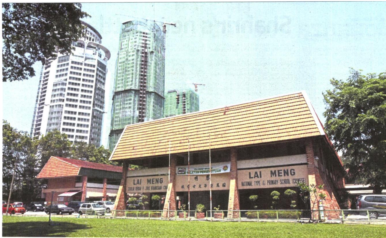
Strategic location: Magna Prima's prized asset is the 2.62 acres that used to house Lai Meng School along Jalan Ampang.
